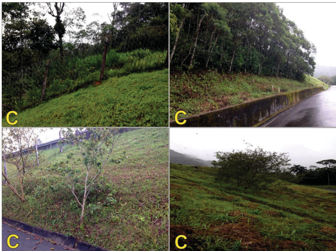
Figure 8: Tilted fences and trees situated on the said slope.
